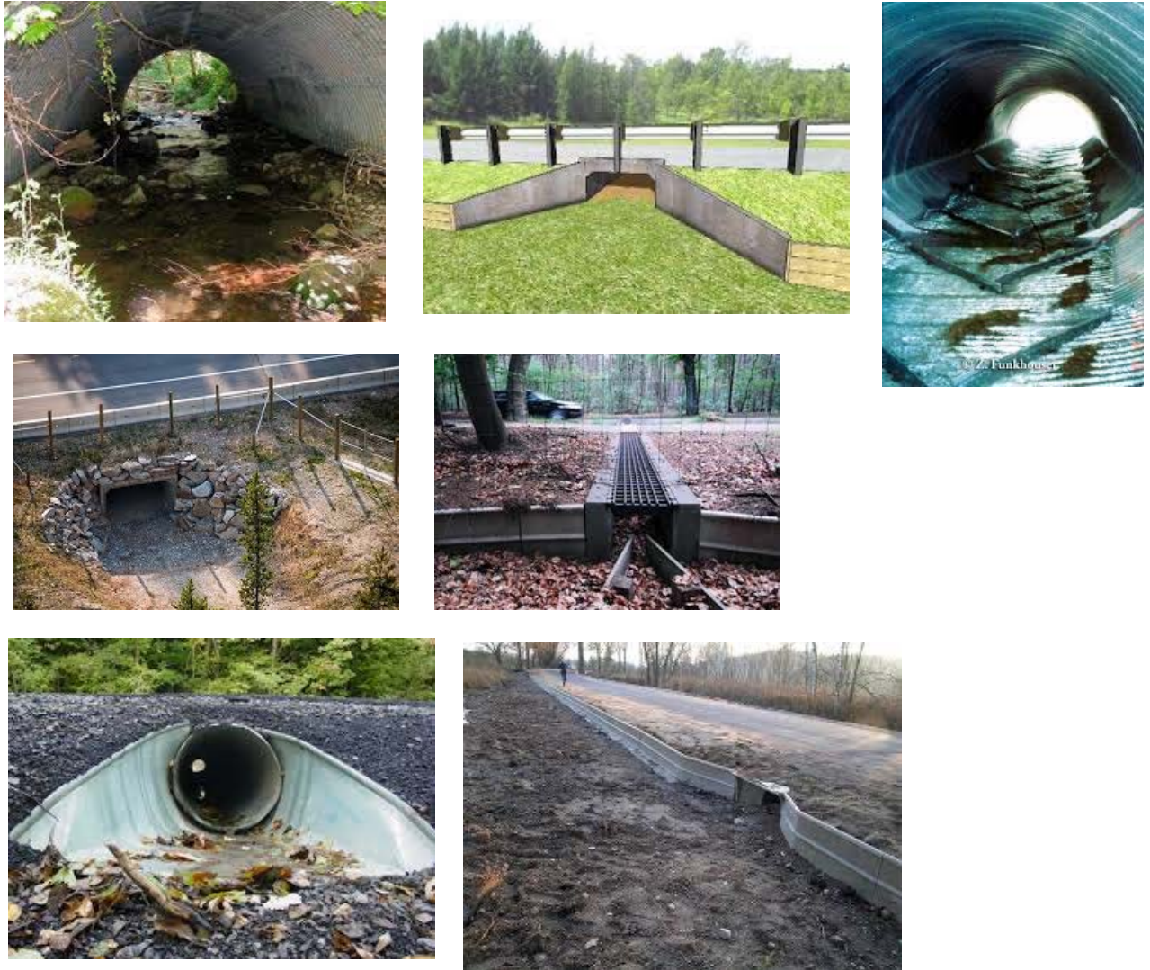
Figure 1: Examples of culverts to allow amphibians and small faunal species to cross roads
