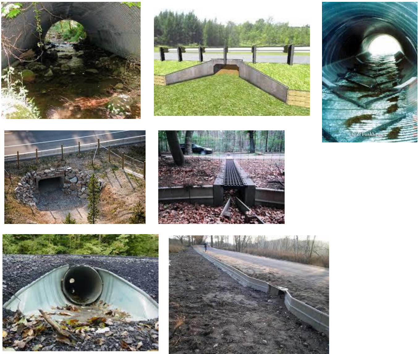
Figure 18: Examples of culverts to allow amphibians and small faunal species to cross roads
