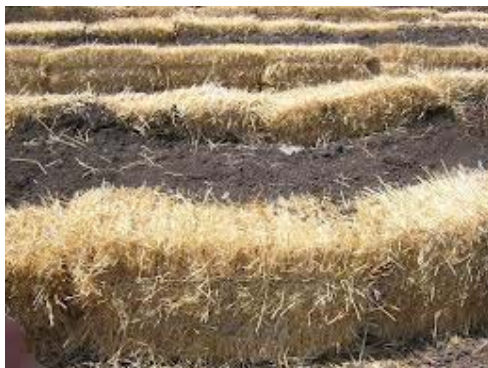
Figure 3: Straw bales must be placed tightly against each other on downhill locations where erosion may occur
